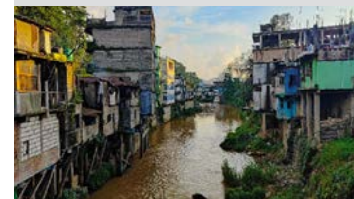
Image 7: Houses constructed on bamboo slits and raised platforms along a stream in Meghalaya; highly susceptible to landslides
