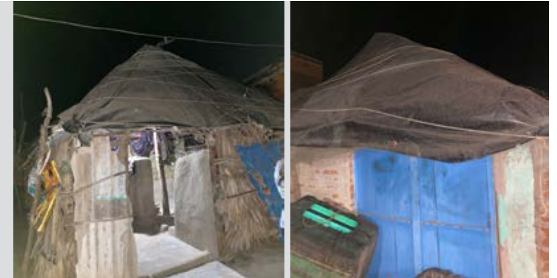
Image 4: Houses of the fishing community (left to right) (a) Roofs are bound together using fishing nets; (b) Roofs being lowered up to 4 ft from the ground
