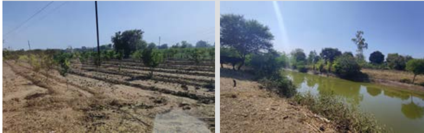
Image 16: (left to right) a) Cement nala bunds; b) Water-harvesting structures built under the Indo-German Watershed Programme in Aurangabad, Maharashtra
