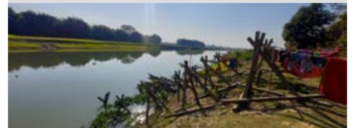
Image 11: Porcupine structures along the river – a traditional remedy to soil erosion
